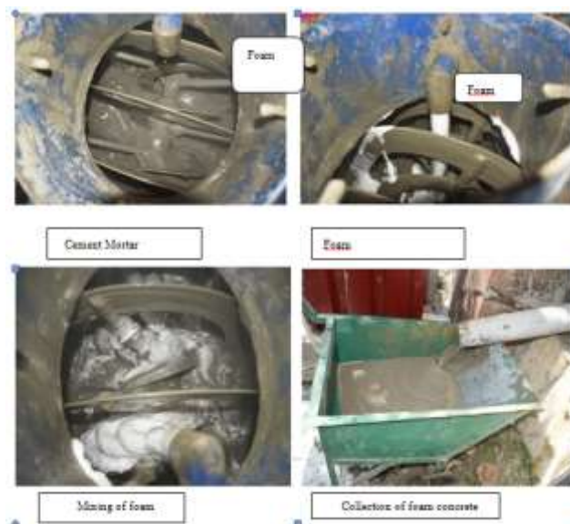
Fig 7 Preparation of foam concrete
