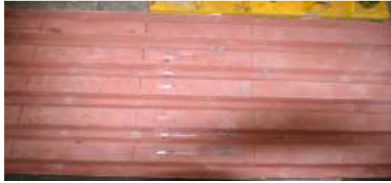
Fig 17 Strain gauge fixed at bottom face of the panel
