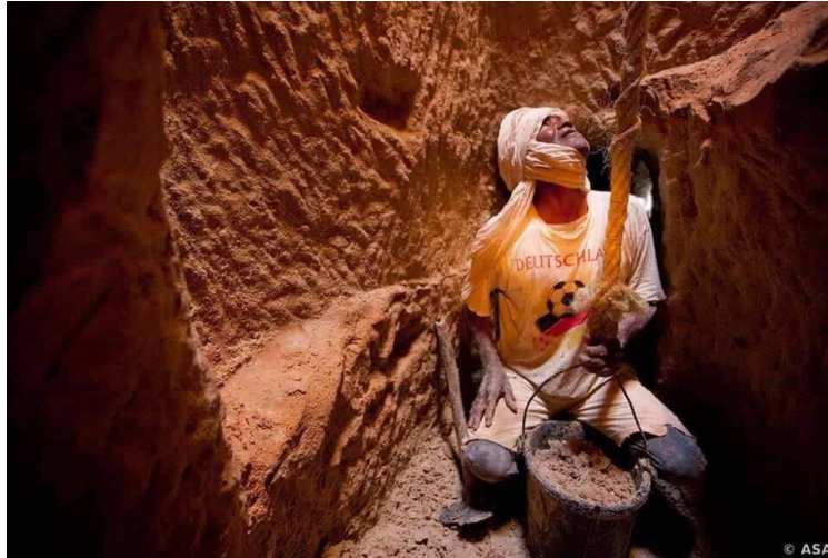
Image No. 01: The excavation process and soil extraction from within Al-Faqra.
